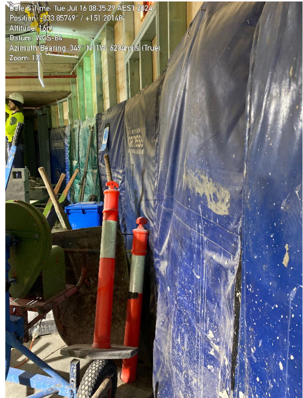
Acoustic blankets lining the internal room currently under construction.
