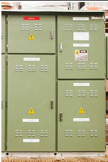
Example of main switch board free standing
