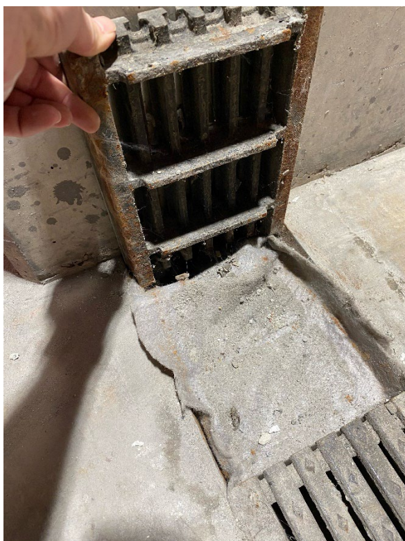
Photo 31 – Geofabric under drain, collecting dust.
