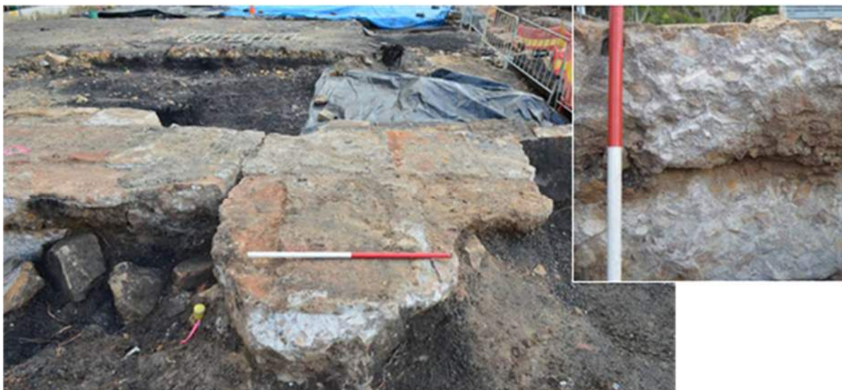
Figure 4.4: Part of the 1880s concrete footing of the Flemish-style building with an inset detail showing the sandstone fragment aggregate. Scale 1m. View to south. Casey & Lowe 2012.
