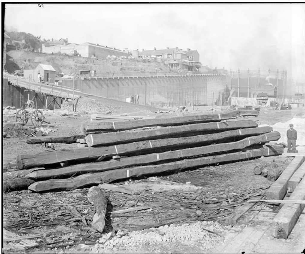
Figure 3.57: Pre-1911 Photograph showing the construction of Hickson Road in the vicinity of the study area, with the Gasworks and large gas annulus visible in the background. SRNSW, 'Millers Point and Hickson Road (Under construction) with Sydney Gasworks gasometer at right', no date, glass plate negative, NRS-9856-3-18-MSBL529.
