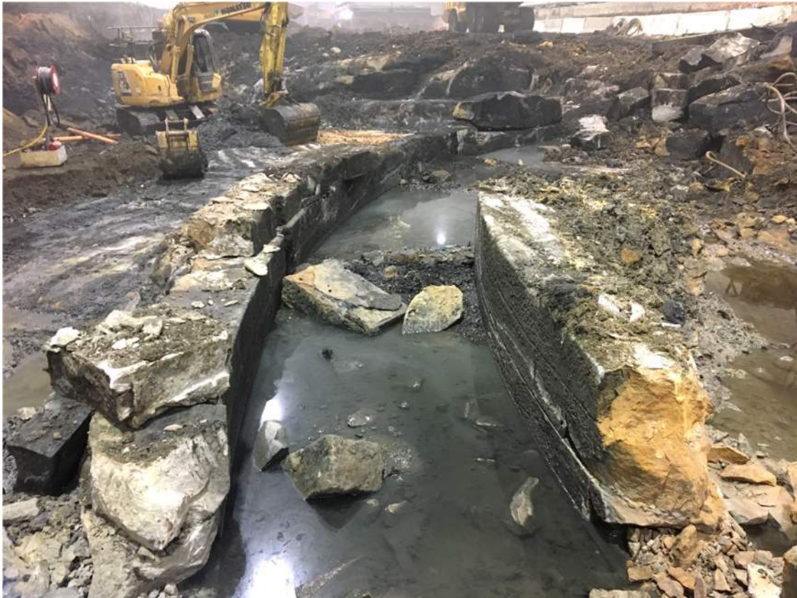
Figure 4.20: Excavation of the 1870s gasholder annulus within Block 4. Lendlease 2019.
