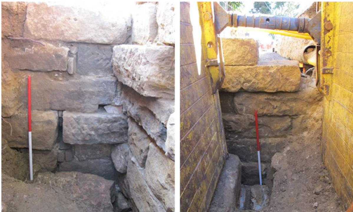
Figure 4.15: Photos showing the depths of the sandstones walls to accommodate the natural topography. The floor in each room dropped in level from east to west from about 400mm to 2.2m below modern street level.
