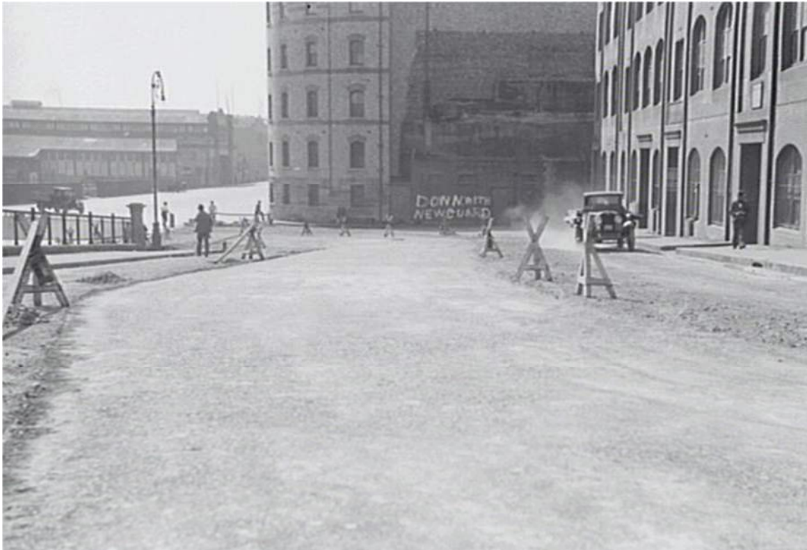
Figure 3.69: Napoleon Street, looking north towards the corner of Sussex Street, 31 August 1932. CSA, SRC8276.
