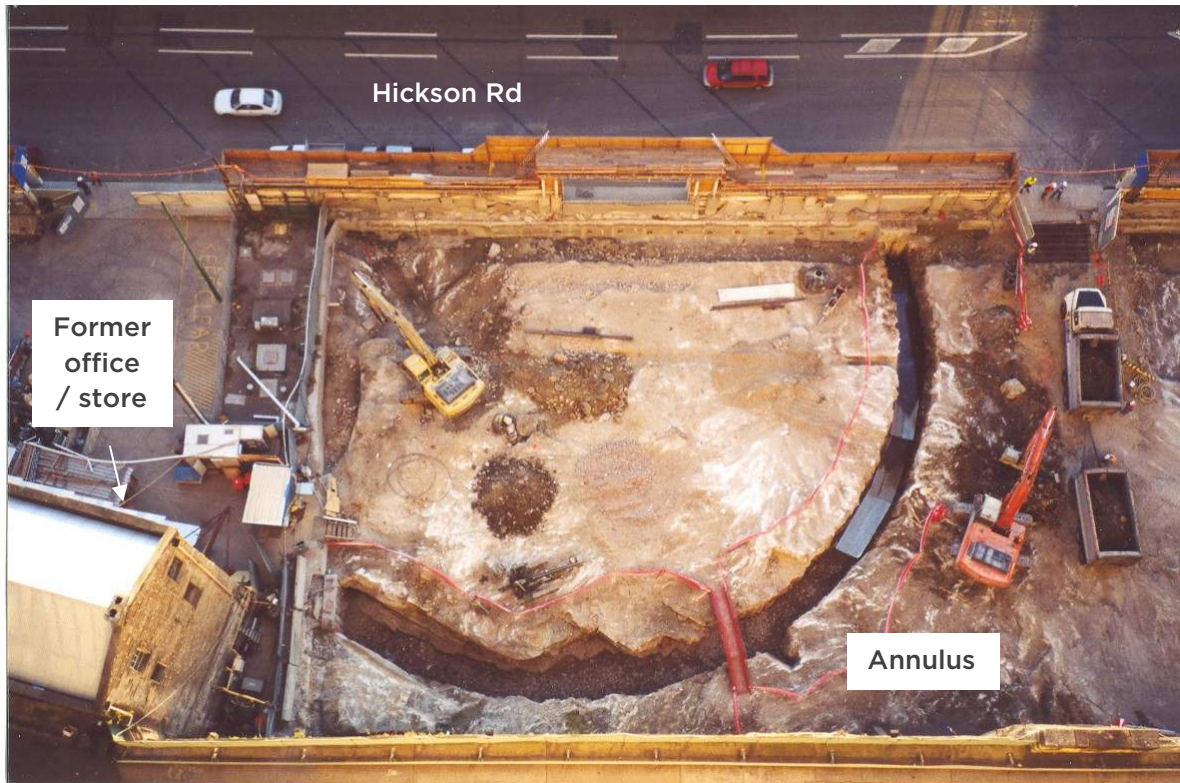
Figure 4.16: Aerial view of the 1882 gasholder annulus recorded at 30-34 Hickson Road, Millers Point (shown to continue under Hickson Road). Image provided by Mark Burns, Lendlease (2002).
