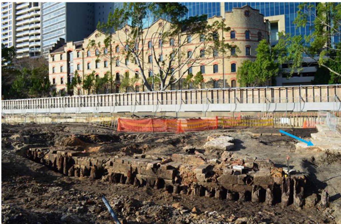
Figure 4.3: In the foreground is part of c.27m of sandstone seawall. On the right (blue arrow) are the concrete footings for the Flemish-style building. In the background is the rebuilt bond building on Hickson Road both part of the Grafton Bond stores. View to northeast. Casey & Lowe 2012.
