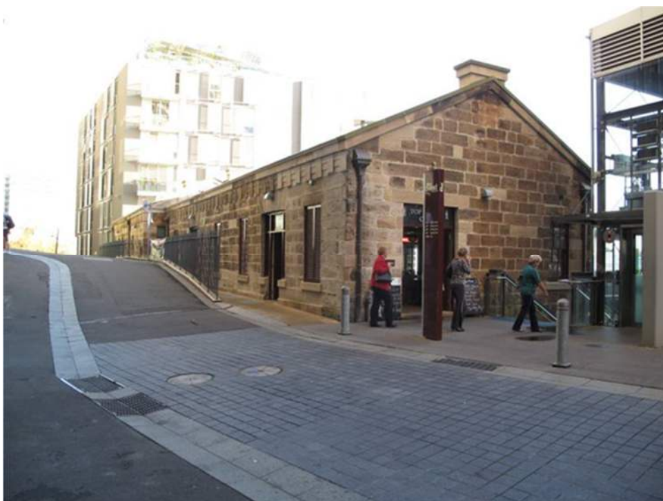
Figure 4.19: Former gasworks building, Jenkins Street above the Hickson Road buildings.
