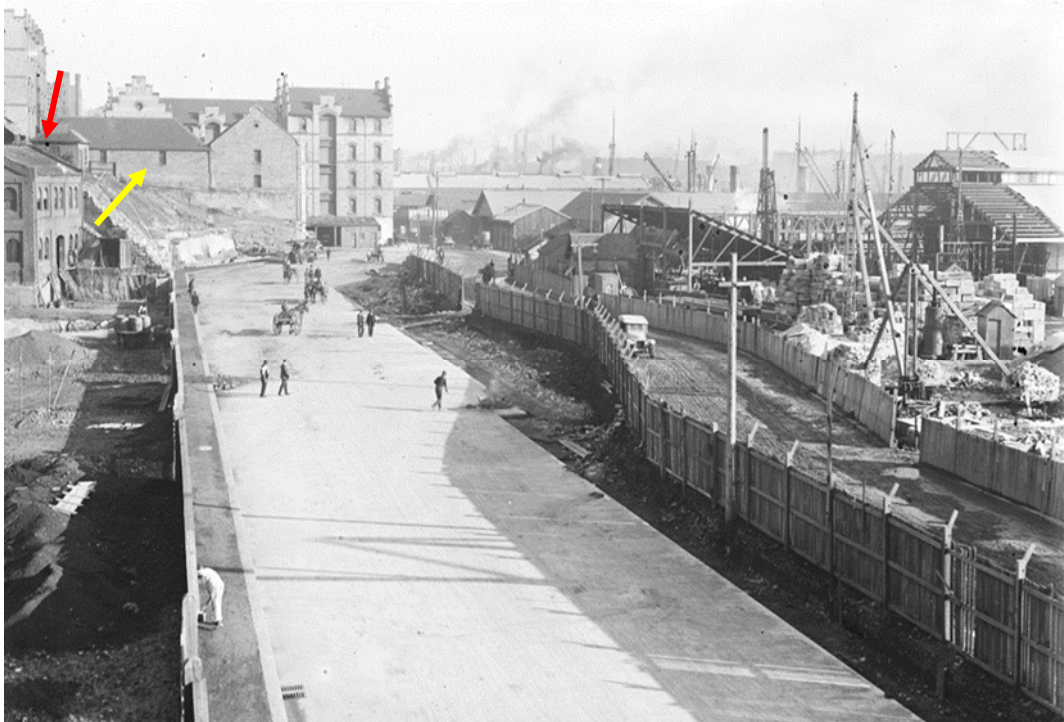
Figure 3.61: Construction of Hickson Road through the former Gasworks site 1923, looking south. Note the front part of the remaining MSB Store Complex building (red arrow). The five-storey building blocking Hickson Road to the south is part of Grafton Bond, soon to be demolished. The 1860s stone store (yellow arrow) built by Smith and Challis, later named Store F. Only the eastern building was retained and the western building was demolished. Note in the photo how the eastern part of Store F is set into the high rock shelf. The temporary road on the West is shown in use. The adjoining slope was quarried to achieve the modern streetscape. NSWSA, NRS-9856-2-142-6454.
