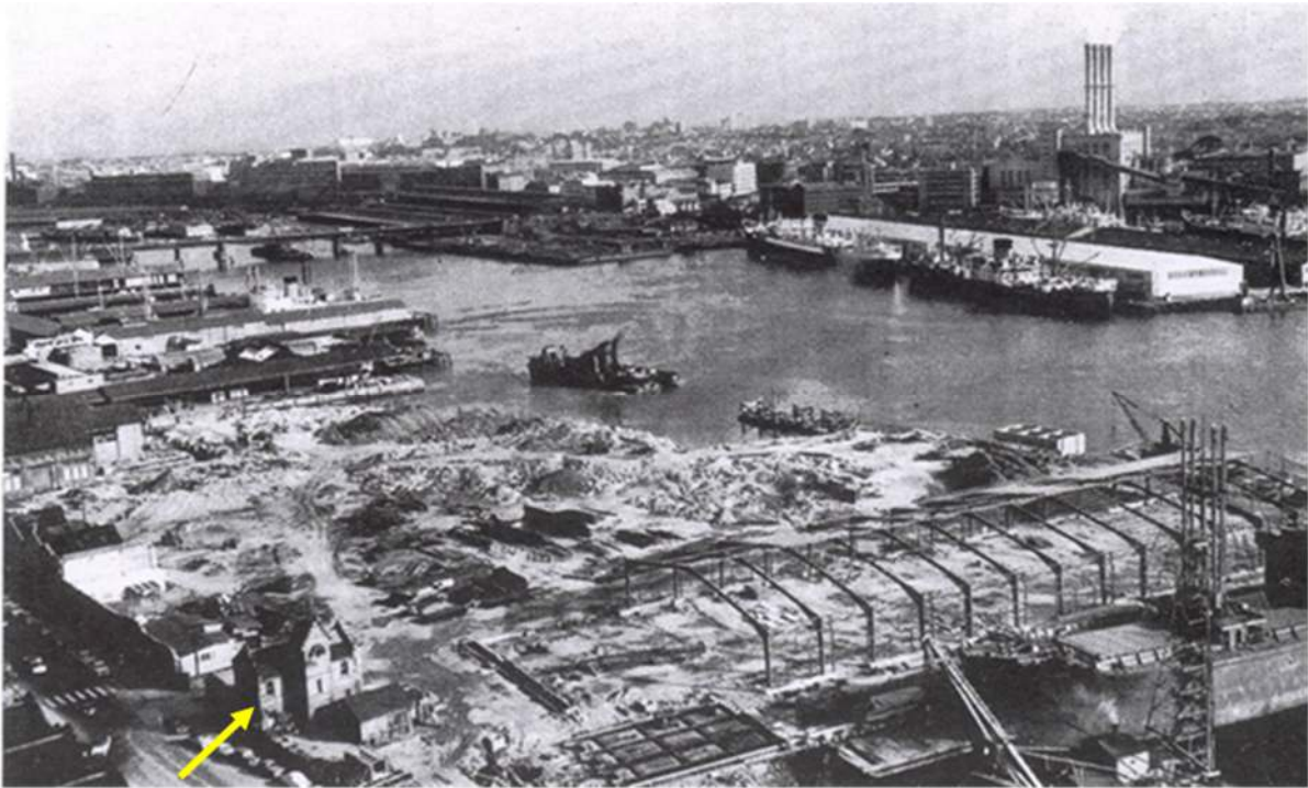
Figure 3.70: 1960s reclamation work in progress on the western side of Hickson Road to create lineal wharfage. Note the small Grafton Wharf tower building in the left foreground (yellow arrow) almost opposite the current study area. Maritime Services Board 27th Annual Report for year ended 30 June 1962.
