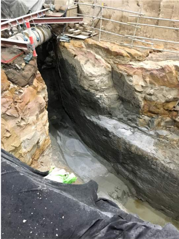
Figure 4.22: The 1870s gasholder annulus within Hickson Rd, cut into the bedrock. Lendlease 2019.
