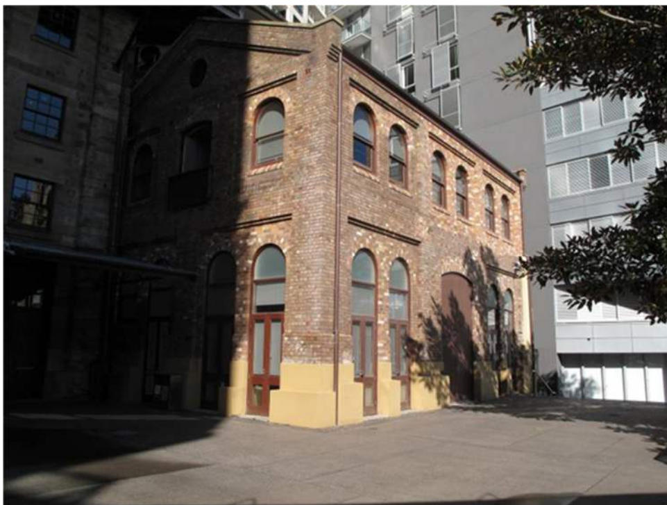
Figure 4.18: Former gasworks building at 36 Hickson Road.
