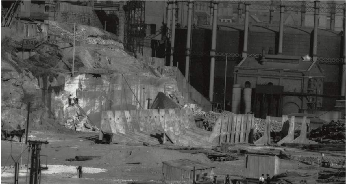
Figure 3.56: Detail showing extensive bedrock modification to the north of the AGL Co Gasworks and the large gasholder, probably associated with the construction of Hickson Road. SRNSW, 'View of the reconstruction of Darling Harbour from Millers Point showing Dalgetys Wharf No. 1 partly completed', 01/01/1909, 9856_a017000007.
