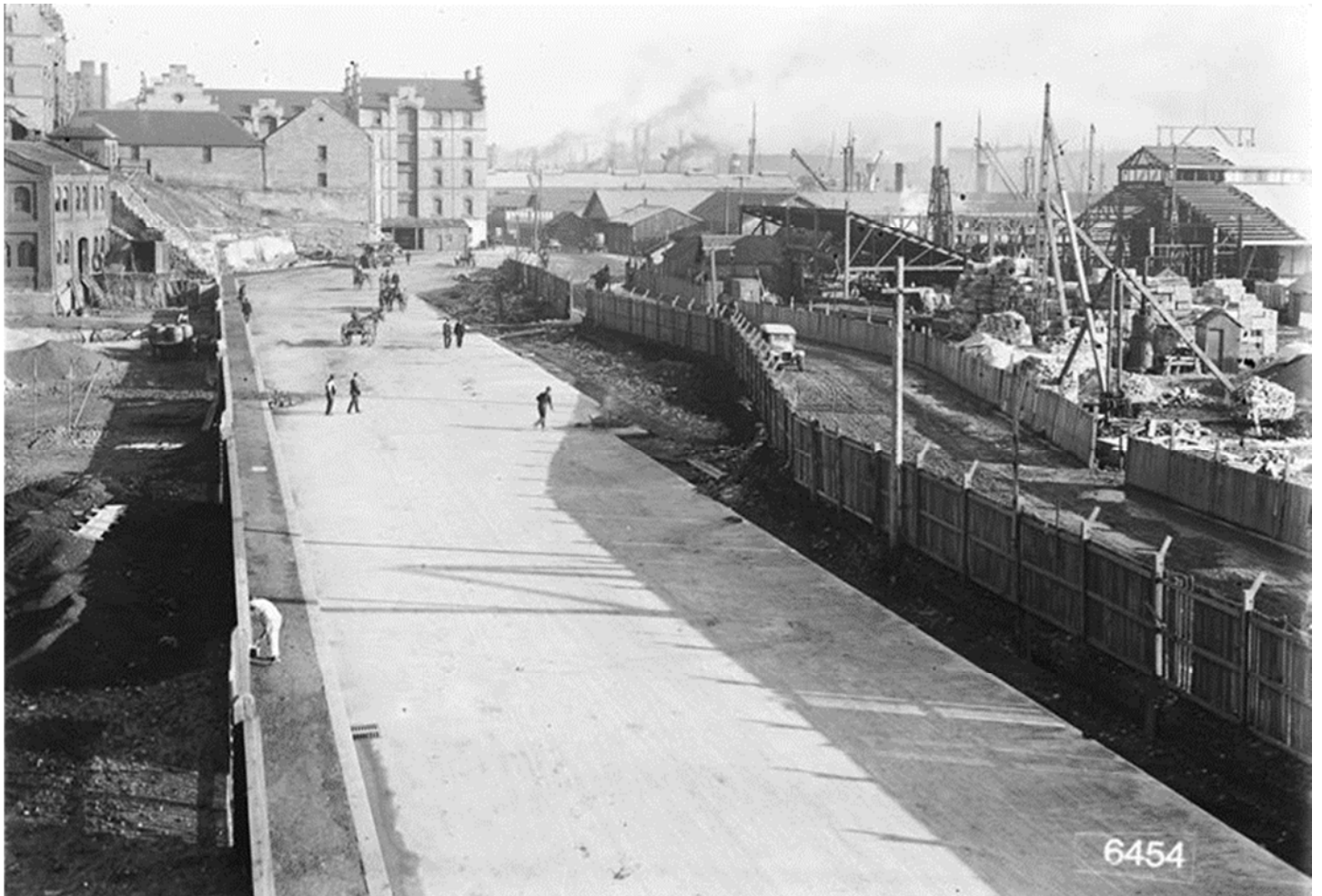
Hickson Road in 1923 after the demolition of the gasworks site, looking south. The five-storey building blocking Hickson Road to the south is part of Grafton Bond, soon to be demolished. NSWSA, NRS-9856-2-[Glass Neg Box1521]-Glass Neg Box 1521-1.
