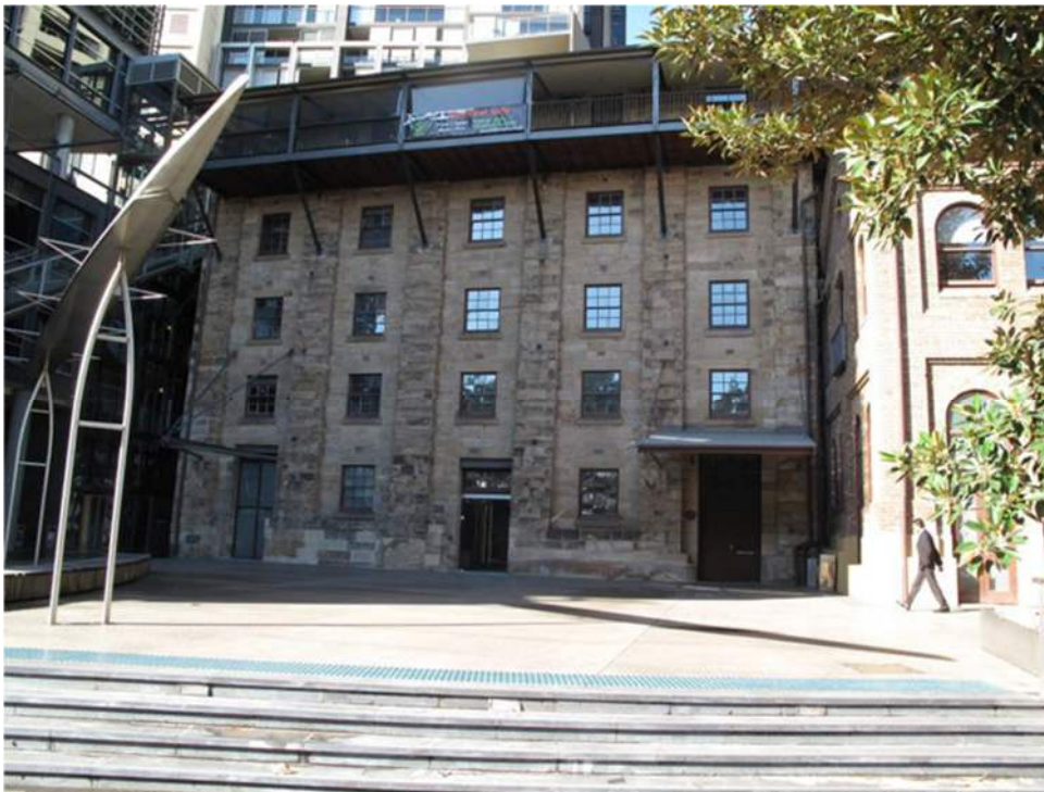
Figure 4.17: Former gasworks building at 34 Hickson Road.
