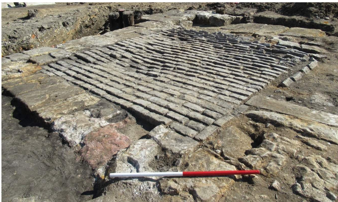
Figure 4.7: Northwest facing view of the termination of Clyde Street showing the bluestone set surface. The surface is orientated with the flow of Clyde Street traffic, suggesting that it was intended for traffic crossing over from Dibbs' northern and southern wharves. Scale is 1m. Casey & Lowe, Preliminary Results Report 2019
