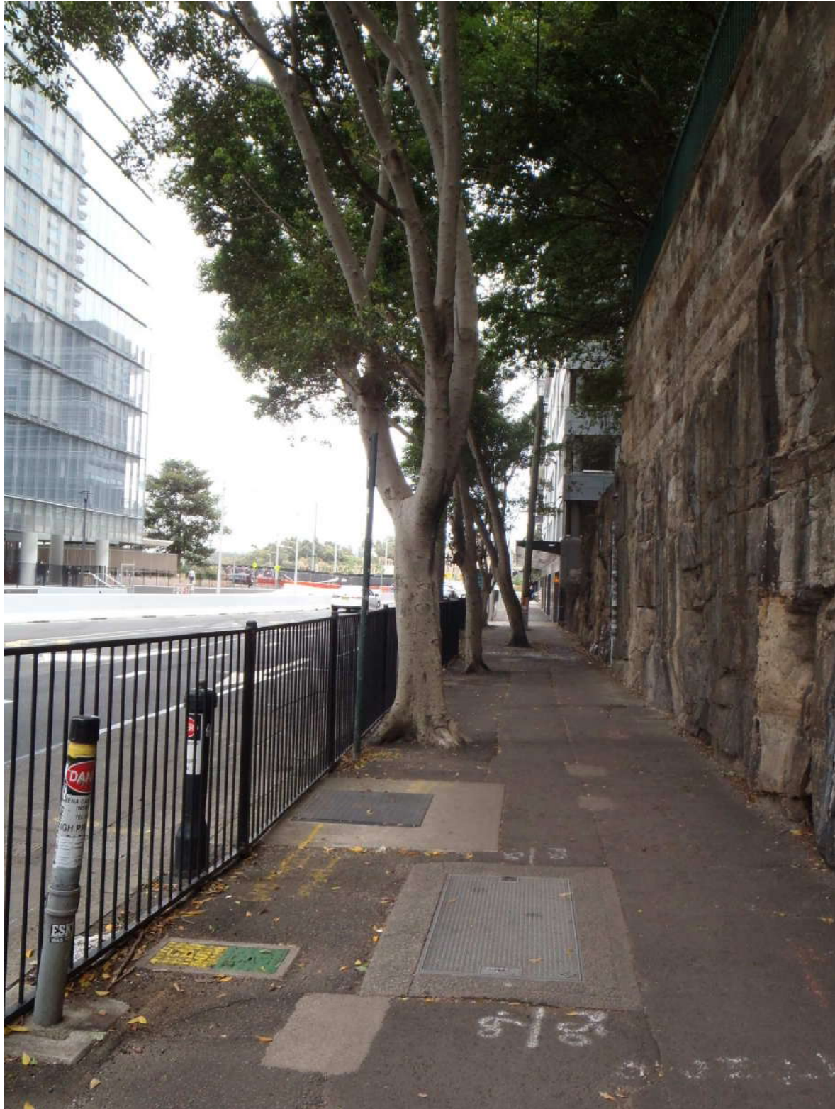
Figure 13. Photo looking north with T11 in the foreground. Note the many underground services and bitumen pavement that is to be upgraded to granite sets with permeable flexible pavement system such as Stoneset © around the Hill's Fig trees (T11-T13) in approximately 3.8 x 2.8m area and approximately 3.8 x 2.1m for T14. Date of photo: 28 October 2025. Source: ELKE
