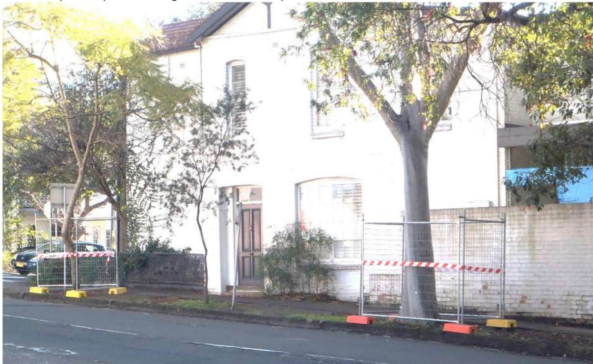
Figure 20 Example of tree protection fencing with pad footings and bolt cleated panels, and TPZ signage.
