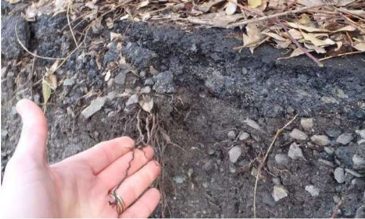
Figure 12. Example photo (not of this site) showing the presence of tree roots within and under bitumen base to illustrate the description and rationale of the recommendations around T11-T14.
