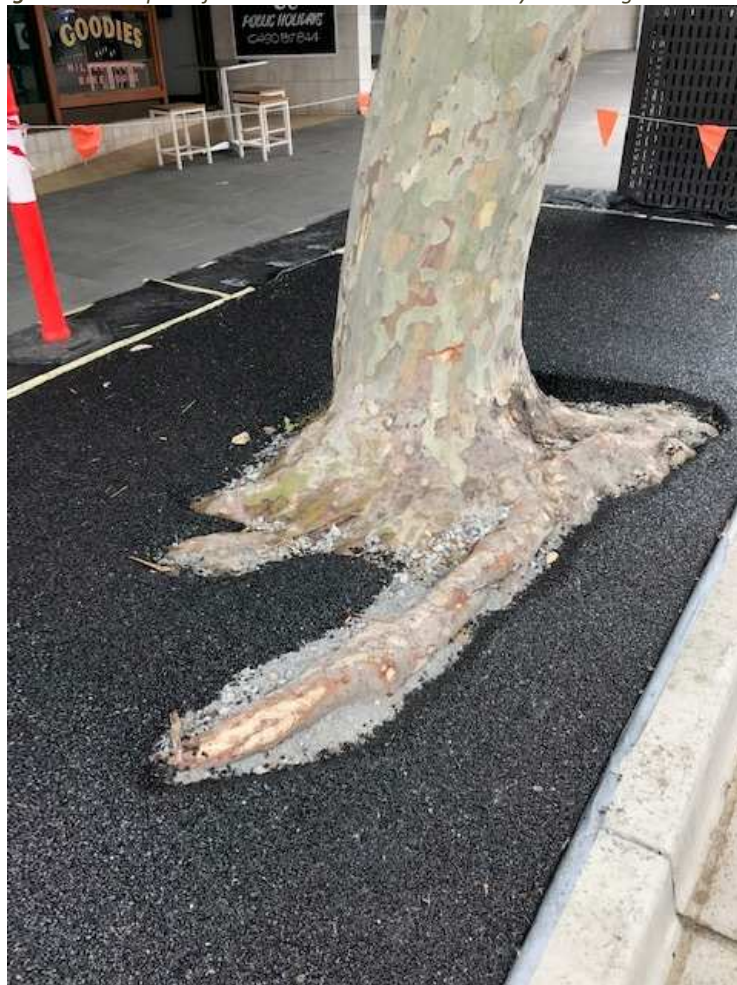
Figure 18 Example image of Filtapave © Permeable pavement System . The above image demonstrates how surface roots are kept exposed where they are above the finished surface level. This is the intent for the Hickson Road South Upgrade Project. Source: Sustainable, Lightweight Filtapave Manufacturers | Sydney
