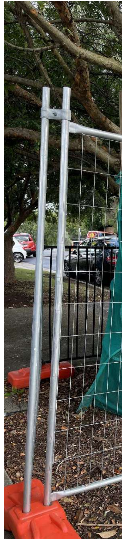
Figure 21. Example (right) of 1.8m high tree protection fencing with pad footings and bolt cleated panels. Example (above) of a TPZ
