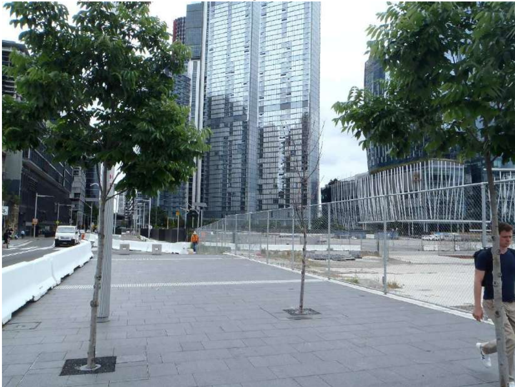
Figure 31 Photos above looking south towards Stage 4 along the western side of Hickson Road. The continuation of the double avenue of Celtis trees is proposed along this zone. Note: the Celtis tree in the centre of the photo has failed (died). There are 3 trees within this newly planted avenue/grove that have died as of 28 October 2025. Date of photo: 28 October 2025. Source: ELKE
